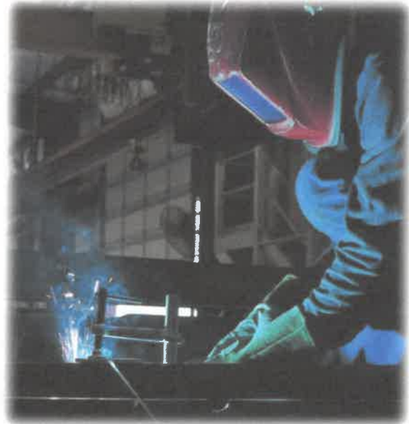
Production Welding in Jeanerette, LA
