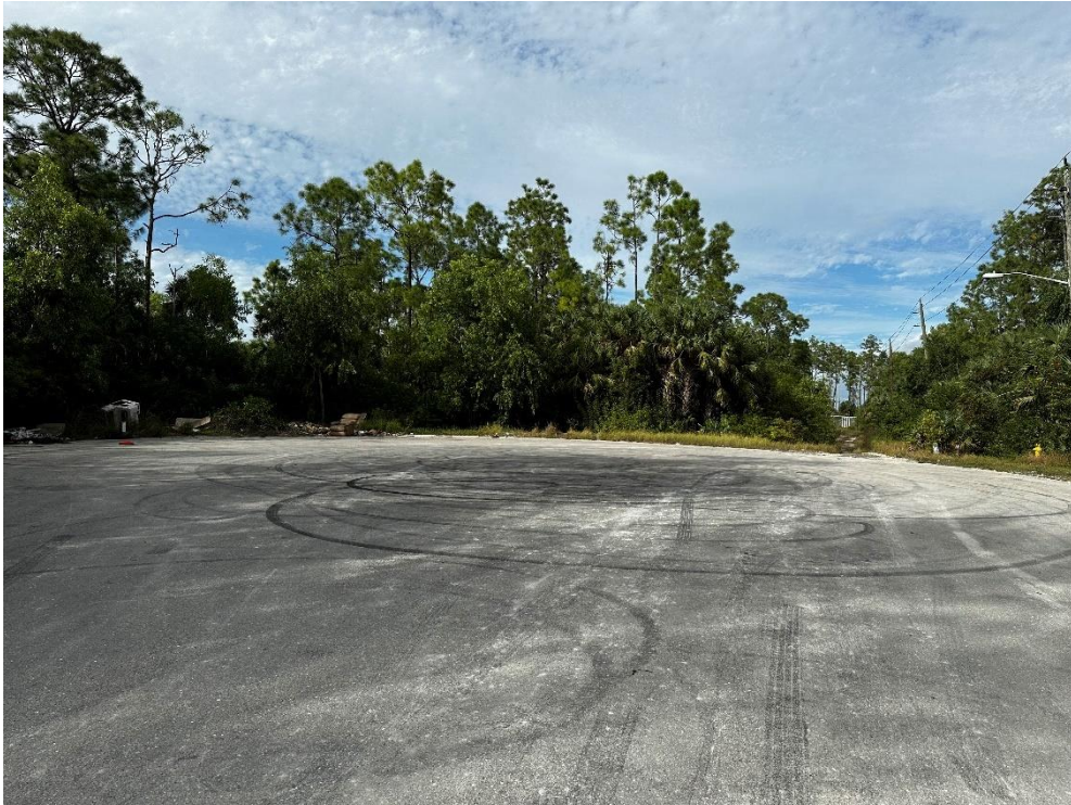
Shearwater Street – Northerly (Photo Taken on December 9, 2023)
