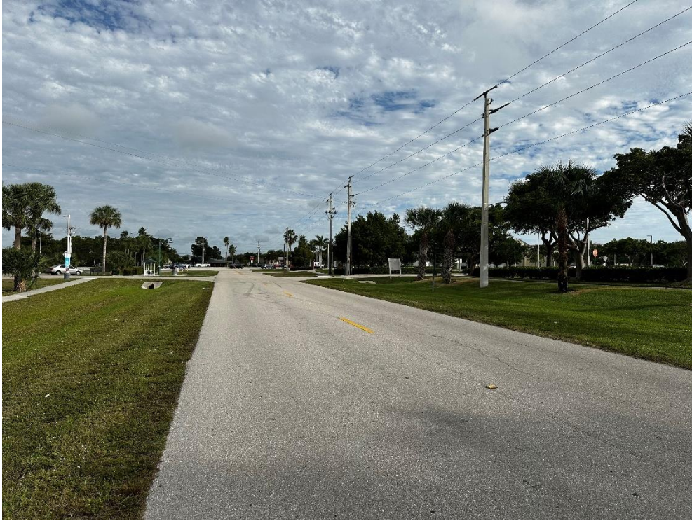
Thomasson Lane – Easterly (Photo Taken on December 9, 2023)
