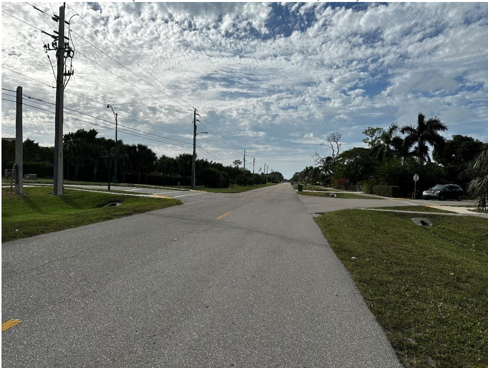
Thomasson Lane – Westerly (Photo Taken on December 9, 2023)
