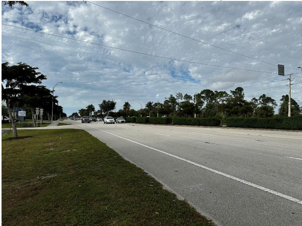
Tamiami Trail E (U.S. 41) – Northwesterly (Photo Taken on December 9, 2023)
